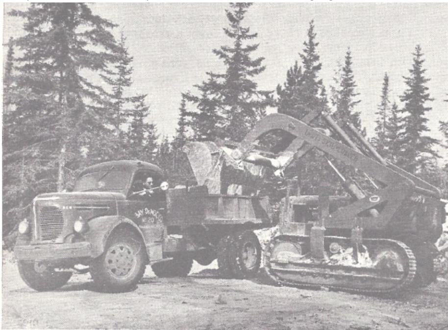
This huge Drott Skid-Loader was used for loading limestone rock in trucks at the American Playground quarry. More than 5,000 truckloads of rock were hauled to the sawmill area shoreline to protect it from water erosion following severe damage to the docks by high water and heavy winds.
